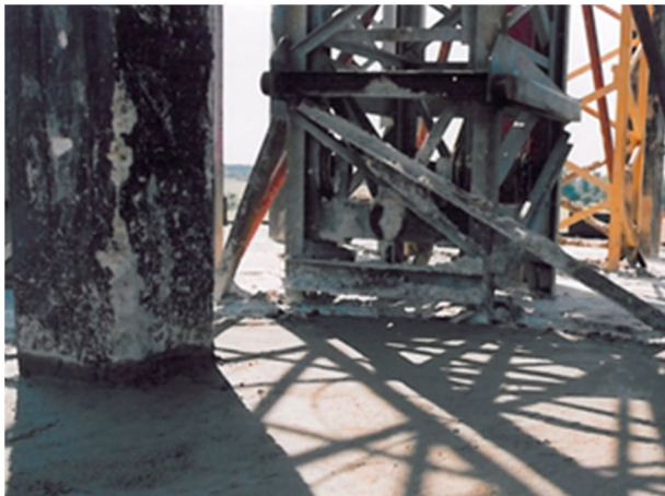
Fig.5. The top plate after concrete casting
